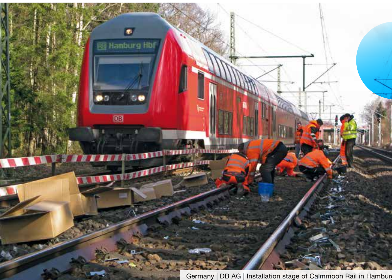
Installing Calmmoon Rail during track possession at night
