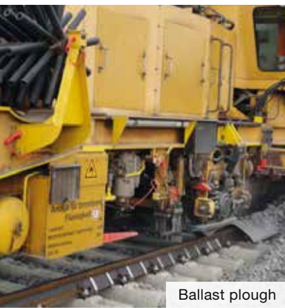
Setting up for ballast tamping
