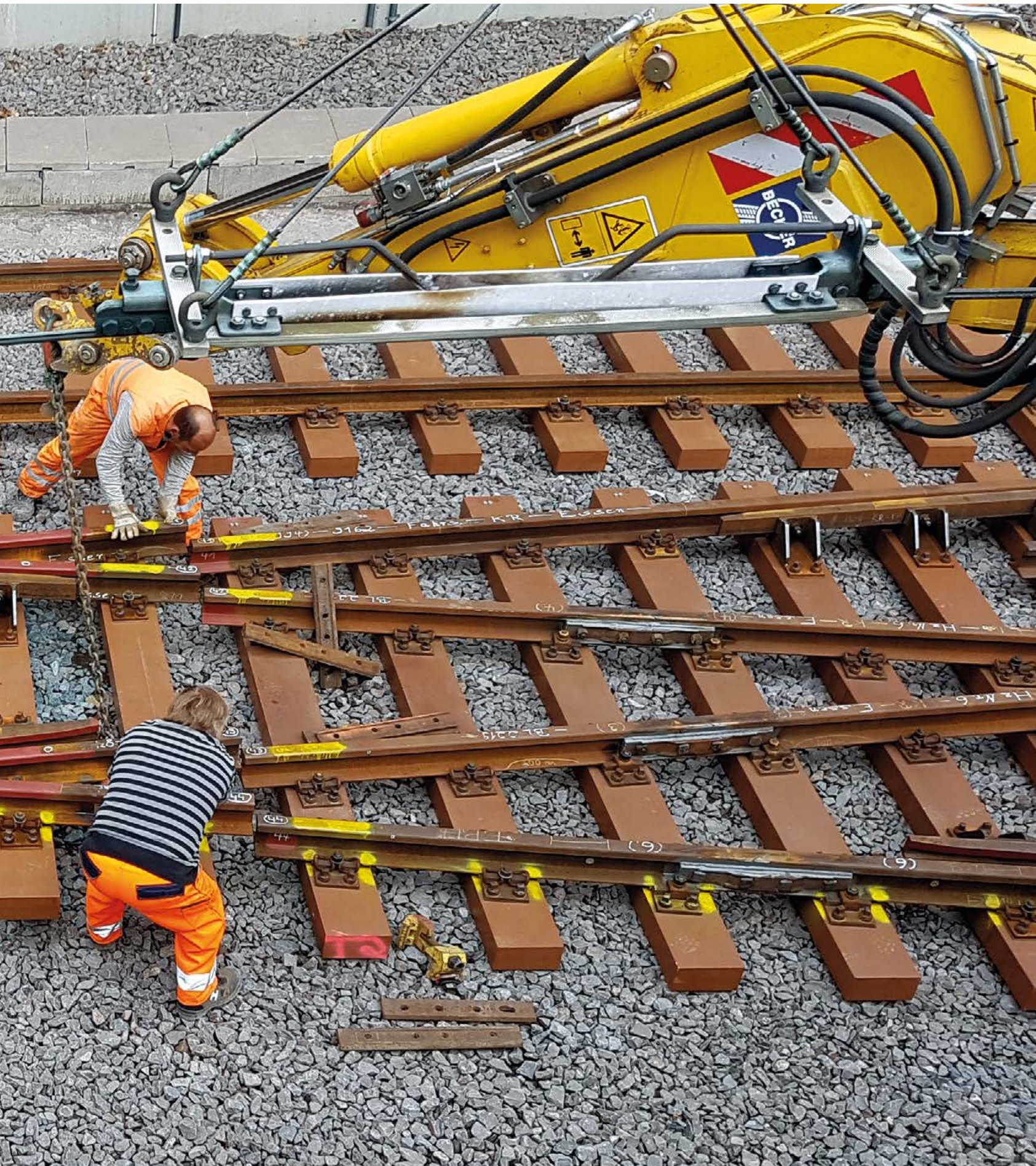
Some of the city railway operators in Germany use FFU Synthetic Railway Sleepers with 10cm height at their switches.
