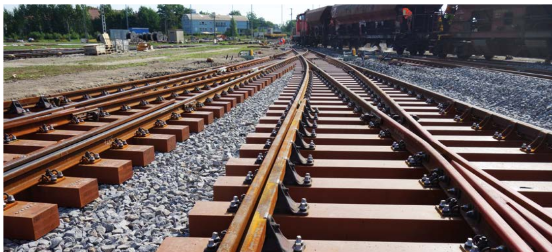
Fig. 1: Deutsche Bahn – Points in the Nuremberg marshalling yard
