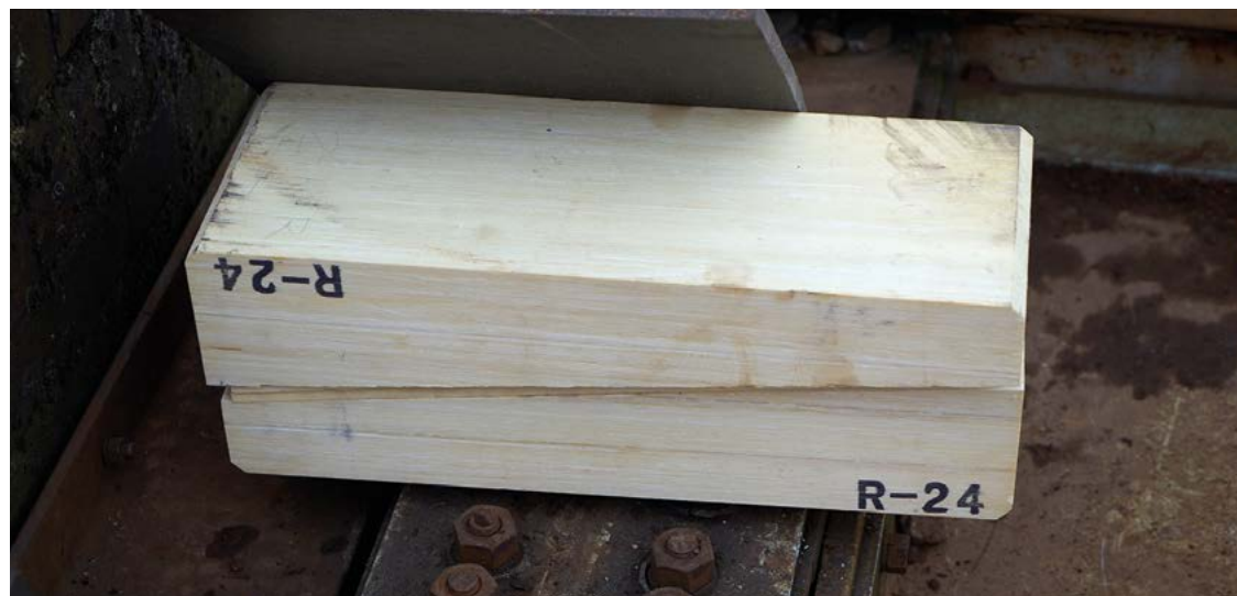
Fig. 5: London Underground Chiswick Park, FFU wedge and layer pads
