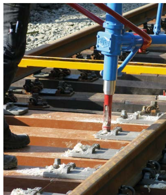
Fig.7: Drilling the holes for sleeper bolts
