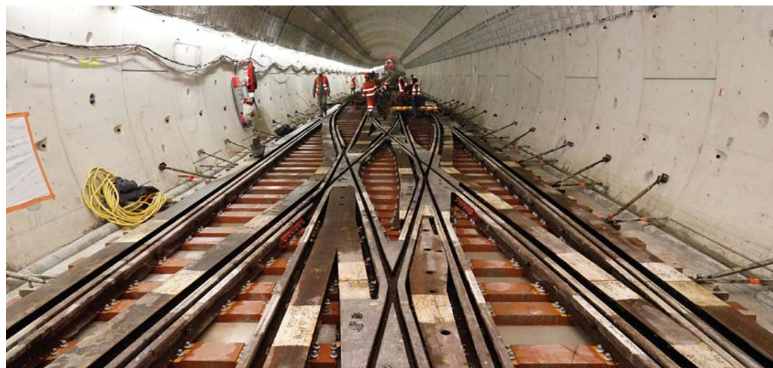
Fig. 6: Paris Metro RATP - FFU in points in the new tracks M4 and M11
