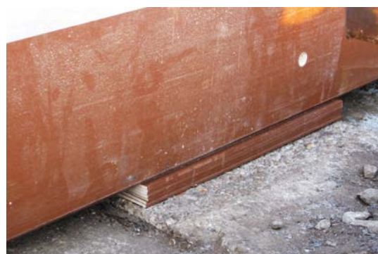
Fig. 5: 3 mm high FFU layers as bearings at abutment wall
